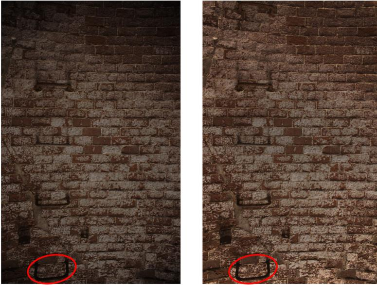
Fig. 12: Result of vignetting correction: Left: The brightness decreases towards the corners of the original image. Right: The metal ladder (red circle) becomes more distinct after correction.
