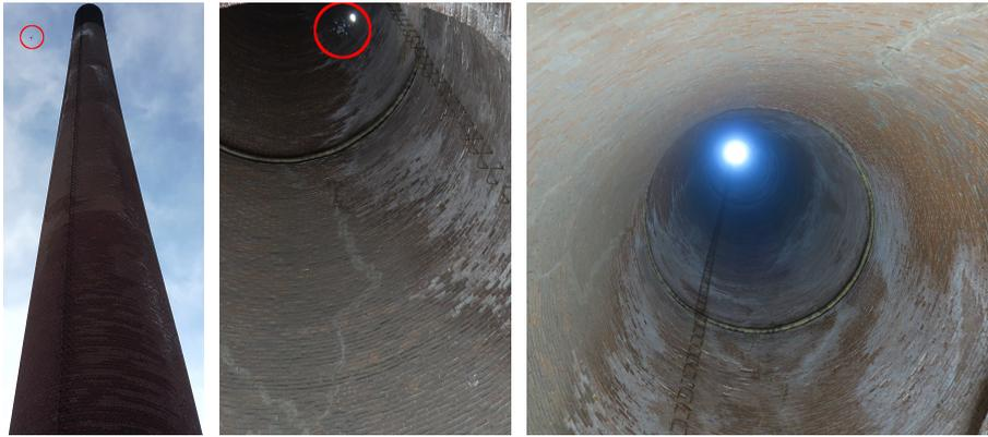
Fig. 1: Challenging flight conditions. The perspective of a pilot on the bottom of a chimney makes flight maneuvers in larger heights hard to control without automation (MAV circled red). Left: Manual chimney inspection from the outside in larger distance from the wall is not suitable for 3D surface reconstruction. Center: Autonomous flight close to the walls. Right: Manual operation in larger heights inside the chimney is prohibitive, especially in daylight conditions.
