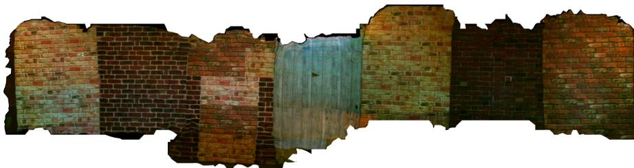
Fig. 14: 2D visualization of the chimney walls. Reconstructed surface of seven walls from the mock-up chimney shown in Fig. 2. Despite some warping effects caused by the unwrapping of the 3D structure, all details are accurately reconstructed.
