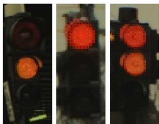
Fig. 6. The color of red and yellow lights might be nearly identical which explains the overlap in the thresholds for the hue in Tab. IV.
